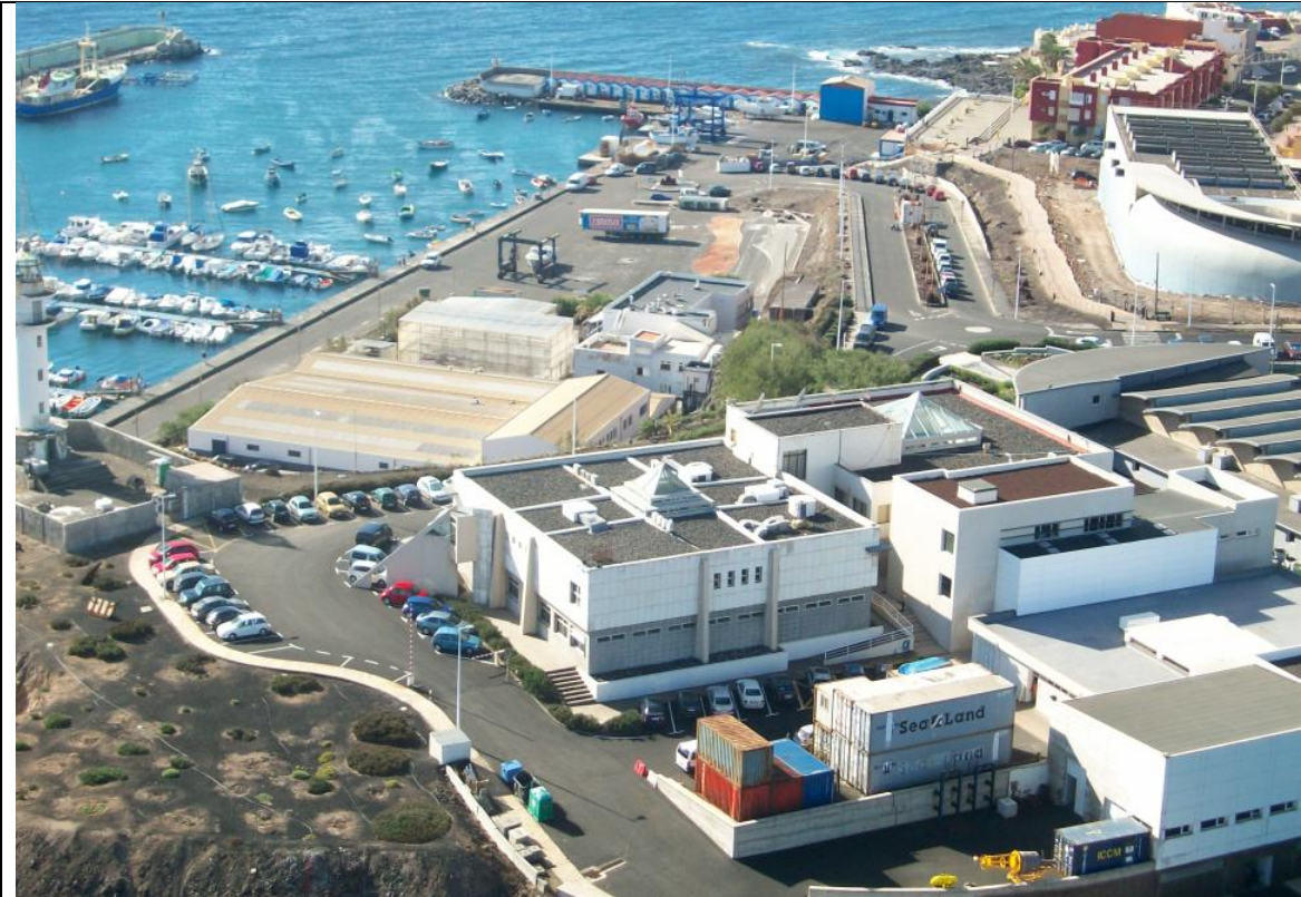
Figure 1 PLOCAN on-shore facilities and harbour pier (Phase 1)
